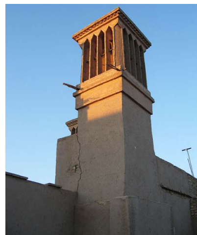
Figure 17. Wind tower in Yazd
