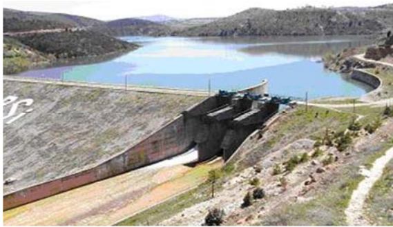
Figure 1. The Kayabogazi Dam [6]
