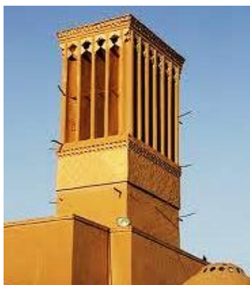
Figure 1. A wind catcher in a house in Yazd, Iran [6]
