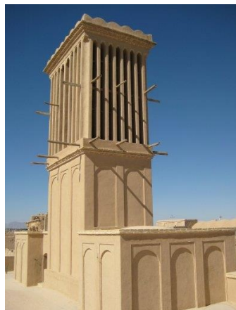
Figure 12. A traditional wind-catcher [8]
