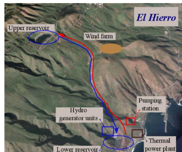
Figure 1. Main elements of the hydro-wind power system
