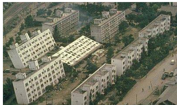
Figure 2. Some effects of liquefaction during the 1964 Niigata earthquake (Photo Credit: National Geophysical Data Center)
