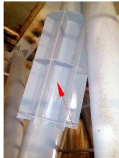
Figure 6. Restored inclined distribution pipe
