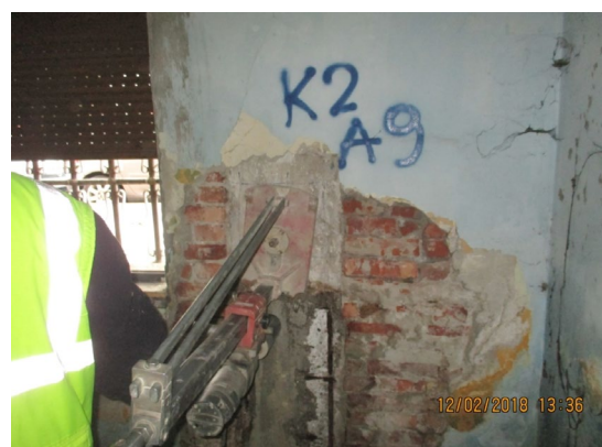
Figure 7. The sampling process at K2 column on Axis A9
