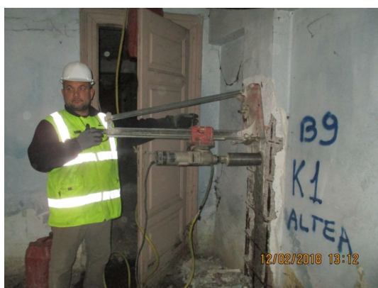
Figure 6. The procedure for extracting a sample from column K1 situated along Axis B9
