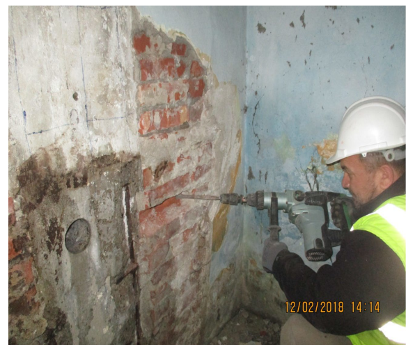
Figure 11. Masonry sample taken from wall, A9
